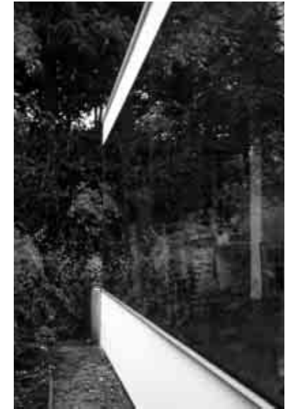
B-House, glued glass façade.
