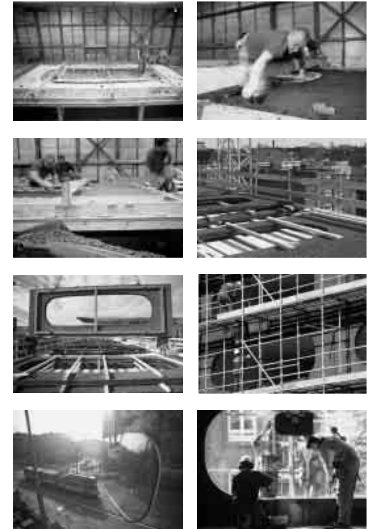
The making and fitting the Sarphatistraat panels.
