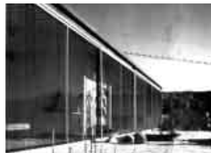
Reference explaining our idea about high-quality outdoor space. The image we used shows the south elevation of the Bailey house, by Pierre Koenig (1959).
