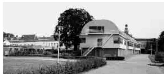
The Clarenburg building without and with the new, almost classical extension.
