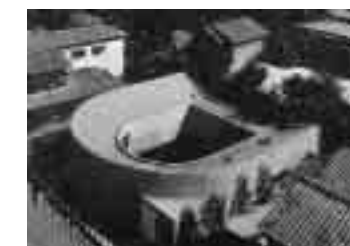
One of the few introvert houses that still offers a view to the world out-side: U-House by Toyo Ito, 1976.
