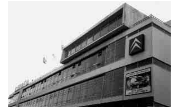
Exterior of Citroën building designed by Jan Wils, adjoining the Olympic Stadium designed by the same architect. The penthouses used to be the canteen of this building.
