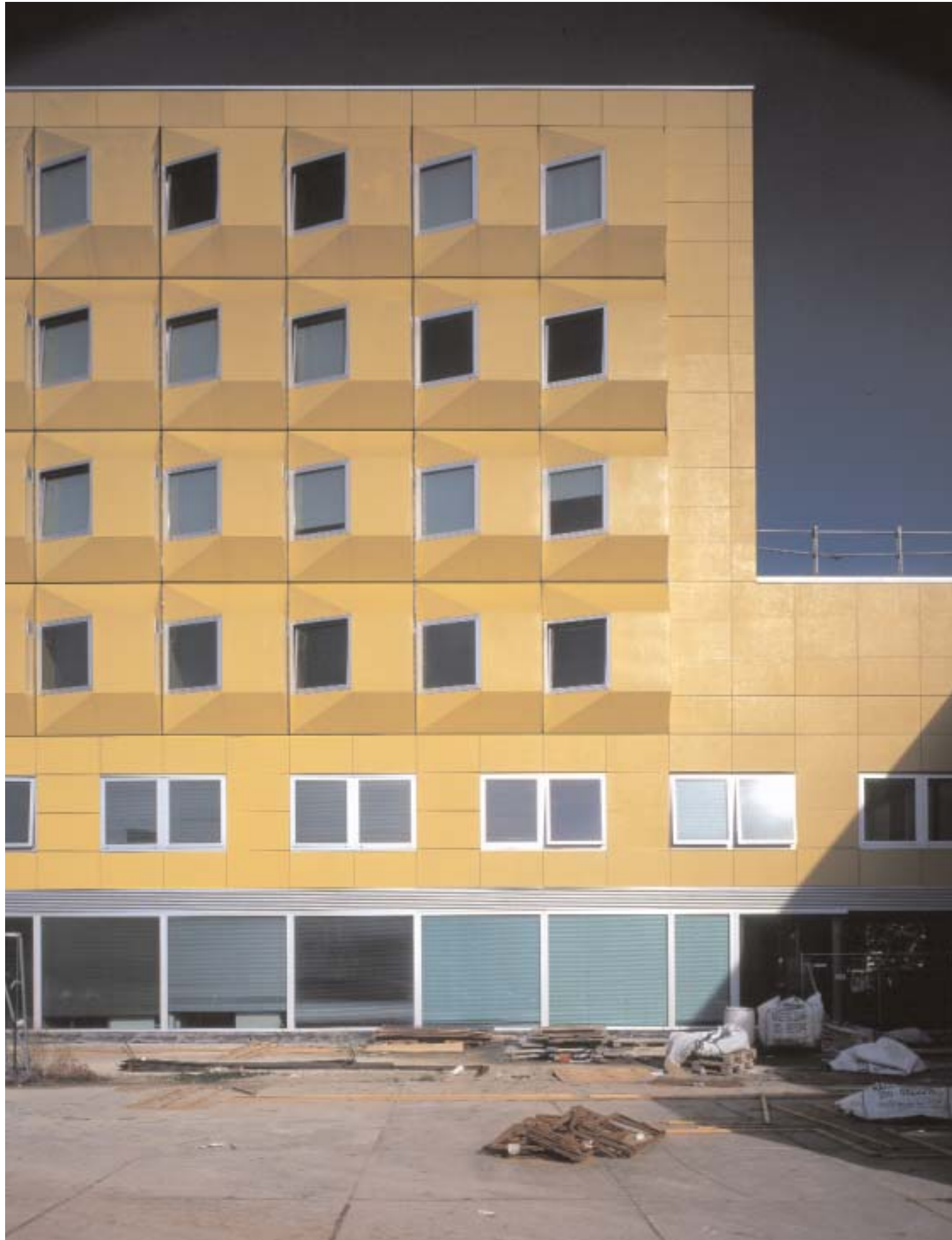
WA-House, urban backland façade, under construction.
