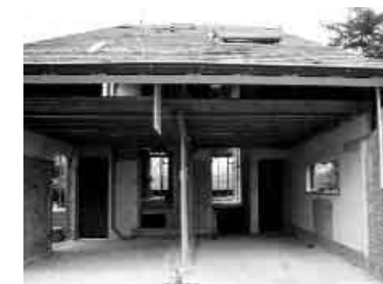
B-House, stripped of almost everything.
