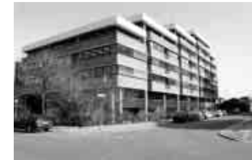
The former office building of Directie Noordzee.
