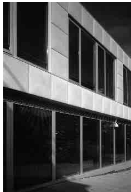
WA-House, civic square façade, under construction.
