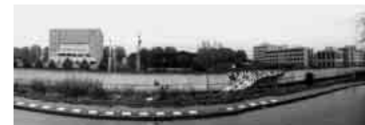
Site seen from one of the neighbouring plots. Site seen from side adjoining the railway line.
