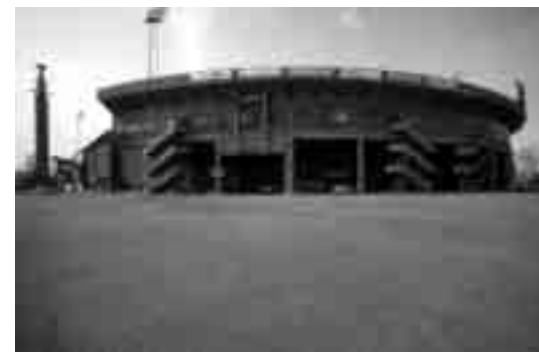
Olympic Stadium, designed by Jan Wils for the 1928 Games. The concrete ring on top of the brick building that was also designed by Wils in 1937 is clearly visible.
