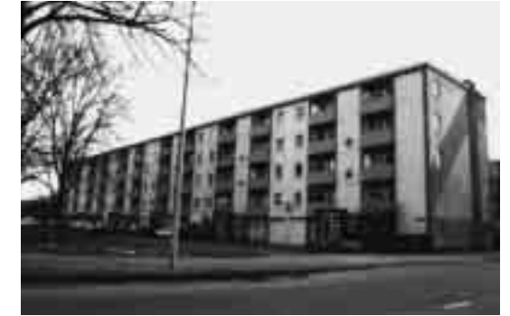
The existing building blocks that we were asked to renew.
