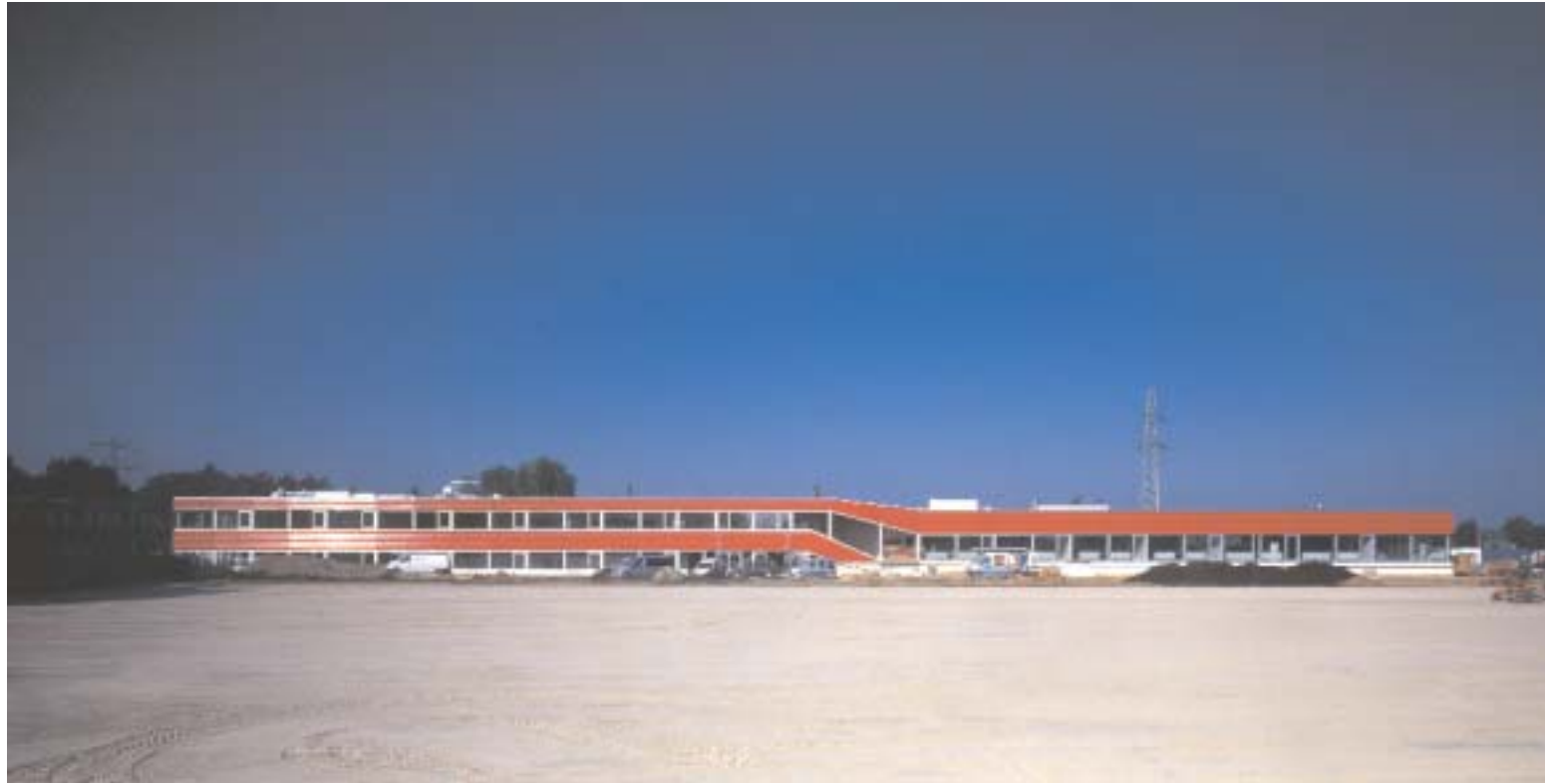
The school in Echt, under construction.
